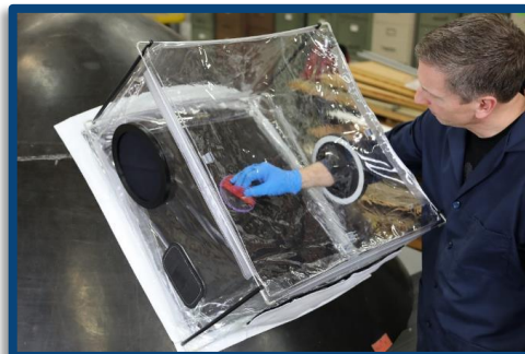
Conform to Repair Site
